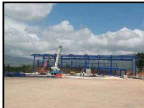
Construction of Toll Plaza
