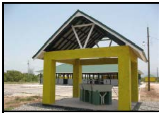
Fish Cleaning Unit
