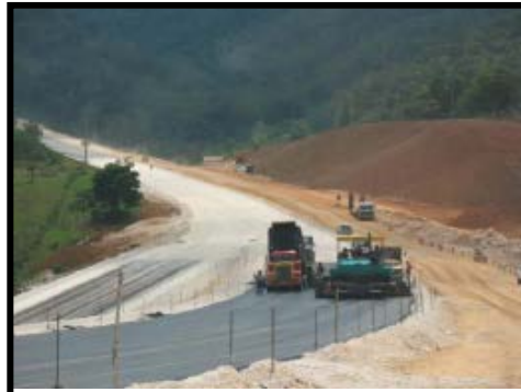
Asphalting in Progress - Km 16+900
