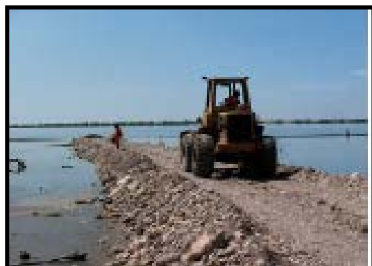
Access road with silt screen in background
