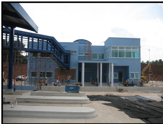
Toll Plaza on Mt. Rosser Bypass
